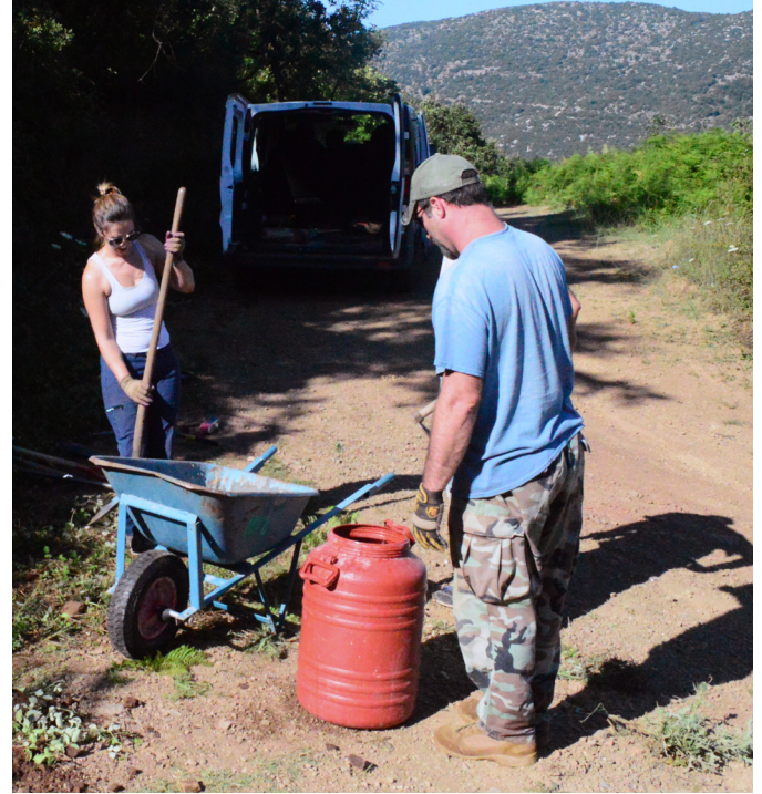
Kelly Moss and John Keck installing new way finding sign on the Trail of Pan
