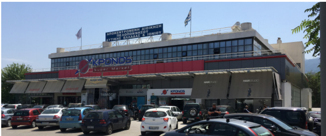
Office building in Patras of Mr. Nikolaos Papatheodorou, Administrative Co-ordinator of the Peloponnesos, Western Greece, and the Ionian Islands.
