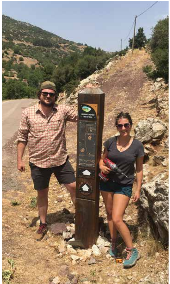
Kyle Mahoney and Lauren Tomanelli doing maintenance work on the trailhead for the Trail of Rhea. Photo: D.G. Romano
